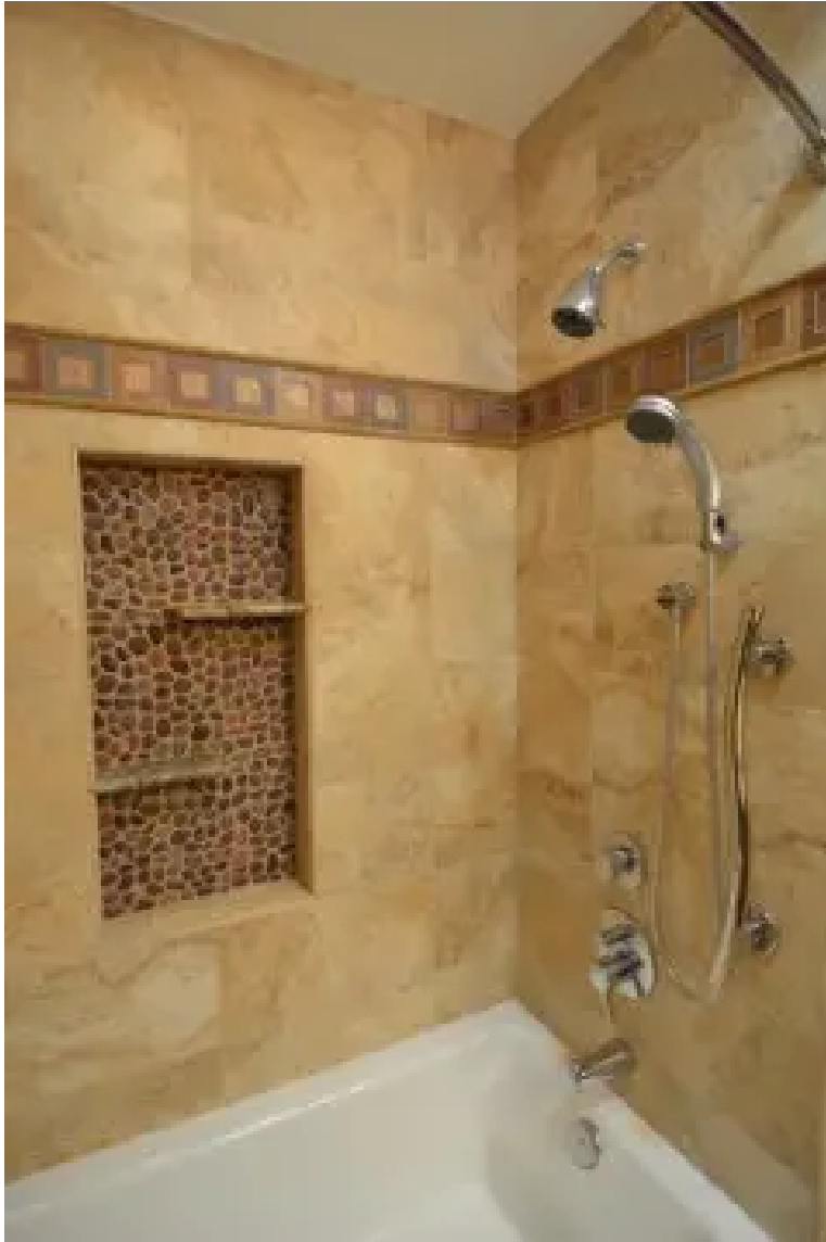
The bathroom is typically one of the most dangerous places in the house. Eighty percent of falls among seniors happen there, according to the Centers for Disease Control and Prevention. Grab bars, color contrasts and textured floor and tub services can help, contractors say. Courtesy of Dan Bawden
